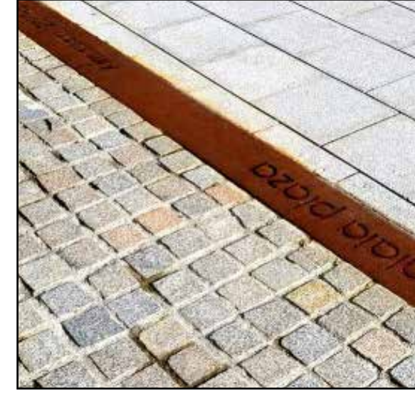
PHOTO: G&C Architects, Landezine, Landscape Architecture Works Granite and Corten 'Rumble Strip' slows cyclists
