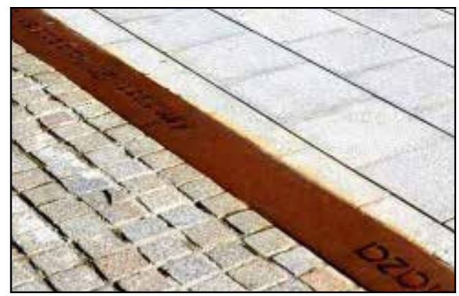
Granite and Corten 'Rumble Strip' slow cyclists
