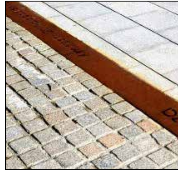
PHOTO: G&C Architects, Landezine, Landscape Architecture Works Granite and Corten 'Rumble Strip' slows cyclists
