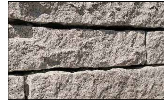
A split-face granite wall will define the plaza
